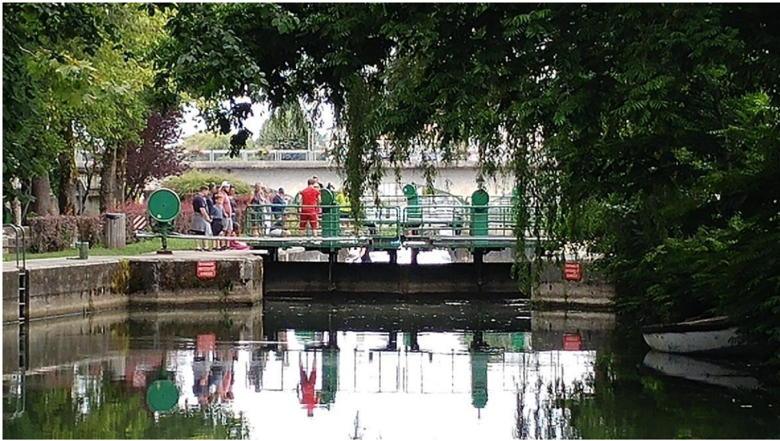
Jarnac Canal (Jarnac Main Bridge Over River Charente In Background)
